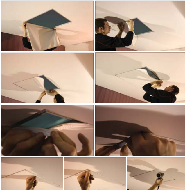
CORNER FIXING WITH TC01
